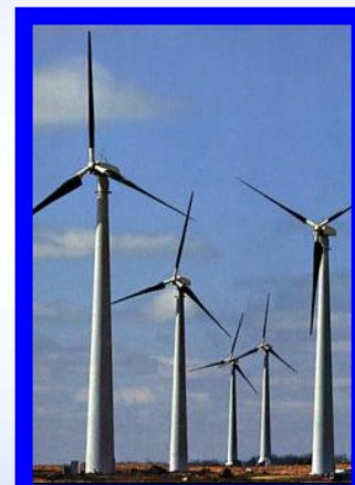
Renewable Energy Generation
